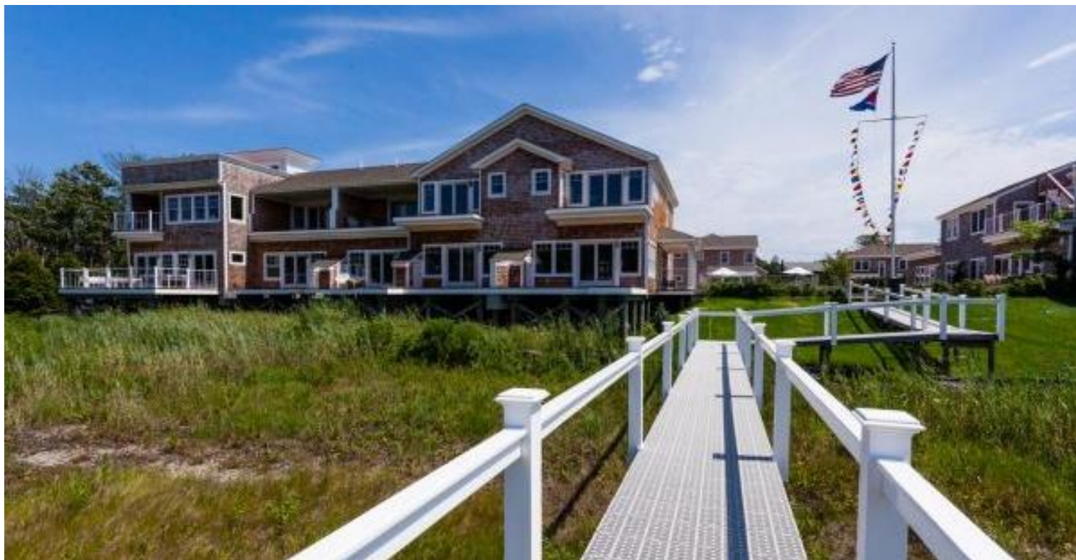
Ponquogue Point, a new private waterfront town house and townhome development under construction, for buyers seeking a second home, on Thursday, Aug. 11, 2016, at 68 Foster Ave., in Hampton Bays. Photo Credit: Heather Walsh
