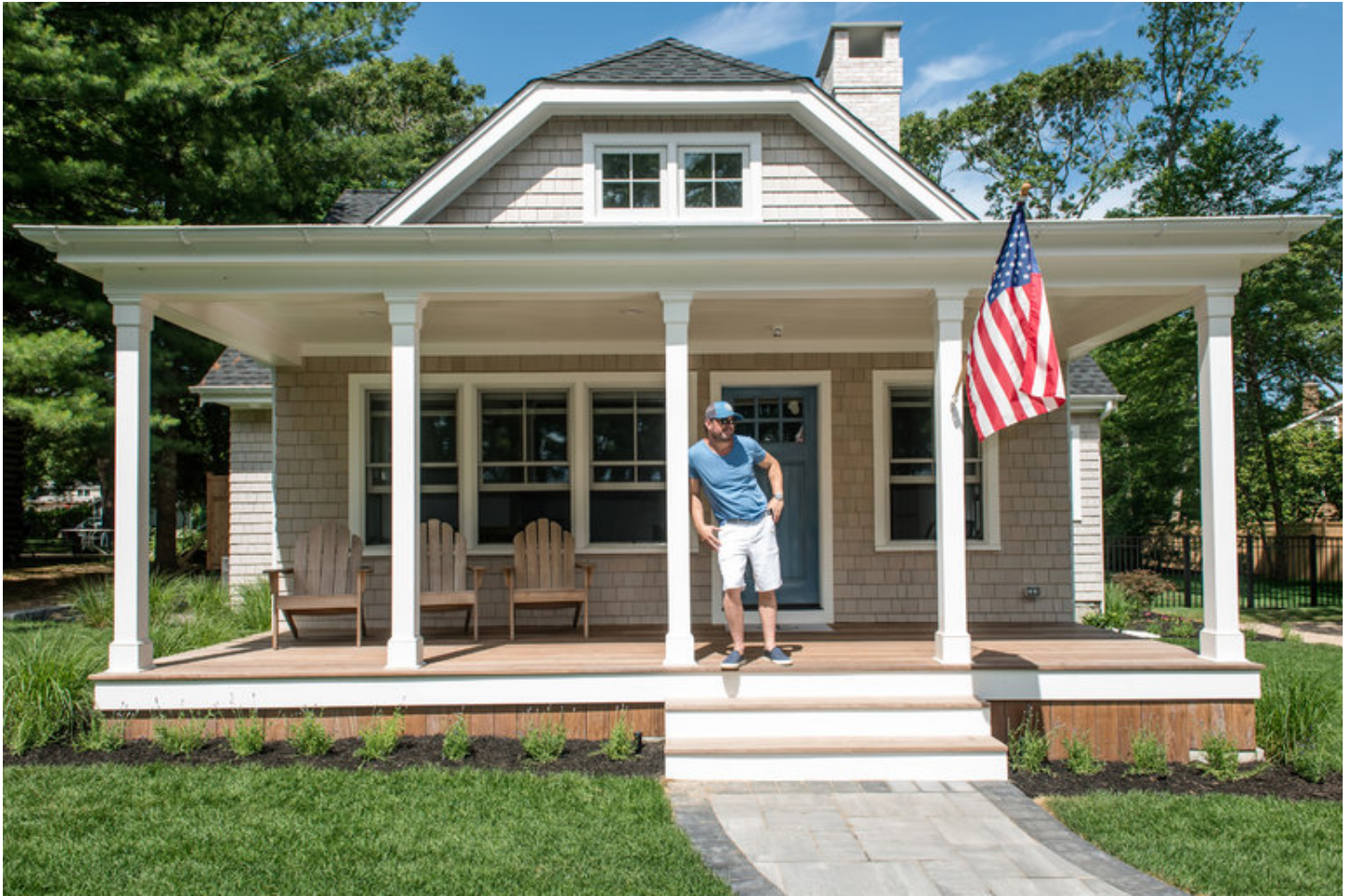
Mitchell Cashwell stands on the front porch of his brand-new bungalow in Southold. Credit Daniel Gonzalez for The New York Times
