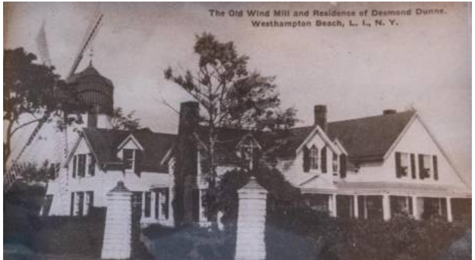
An archival photo of 15 Sunswyck Lane, which was built in 1894 for Desmond Dunne. Credit: Courtesy of Joanie Blagdon
