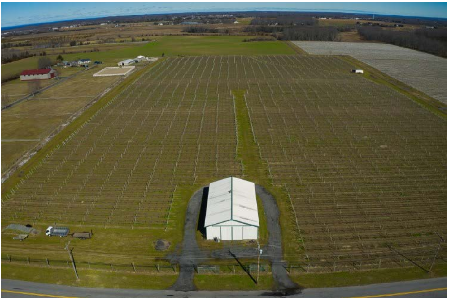
A Morton building, partially finished and insulated, was built in 1993.
